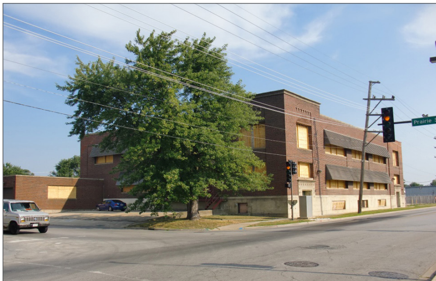
Affected building (above)
